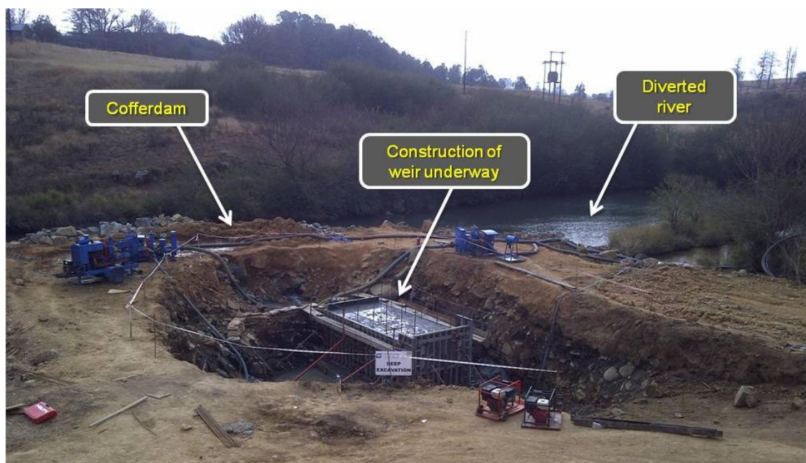
Figure 18: Example of a cofferdam used to create a dry works area
